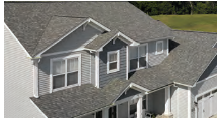
ROOFING AND VENTILATION
