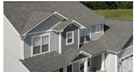
ROOFING AND VENTILATION
