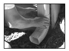
Fit the downspout into the bottom corner, but do not screw it together.
