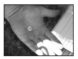
Remove the zip screws you had used to temporarily attach the flip-up. Install SnapLocks to securely attach the flip-up.
