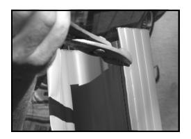
Bend the sides around to make it twice as thick so it will be strong where it is attached to the downspout.
