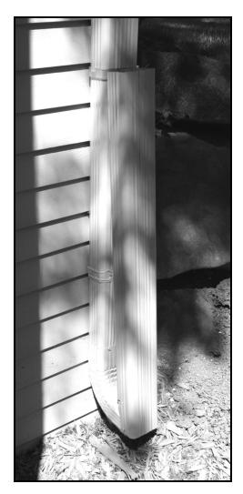
Completed Downspout and Flip-up. While up, the flip-up is ready for mowing and land-scaping, but the homeowner should lay it flat before rain.
