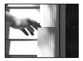
Tip the flip-up up so it meets the downspouts. Make adjustments as needed to the bottom corner so the flip-up lines up with the downspout. Screw the bottom corner into place once everything is aligned.
