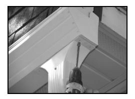
Screw in the Big Mouth and attach corners. Don't over tighten.
