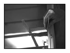
Attach the pipe bands to the siding. Use gutter screws if it is wood siding, use zip screws if it is any other type of siding.
