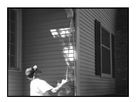
Tack the bottom elbow into place, so you can measure how long of a downspout you will need. Measure from the top of the bottom elbow to the bottom of the corners. Add 3" to your exact measurement so you will be able to tuck it into the corners.
