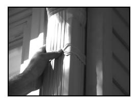
Bend the pipe band around the downspout and screw into place. Do not over tighten.
