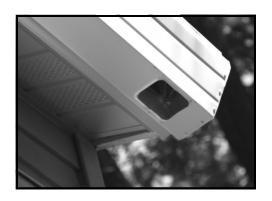
Hold the Big Mouth up to the gutter, and mark on the gutter where the hole in the Big Mouth is.
