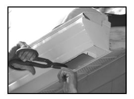
Then, using a tin snip, cut the gutter so the opening is the same as the opening in the Big Mouth.. Bend tabs down and cut to 3/4 inches long.
