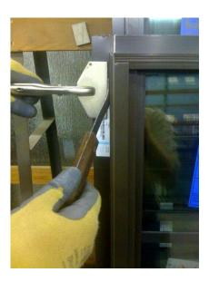
2. After removing the fin, attach the mull strip to the edge of the unit on front and back side of the unit by hand (loose fit)
